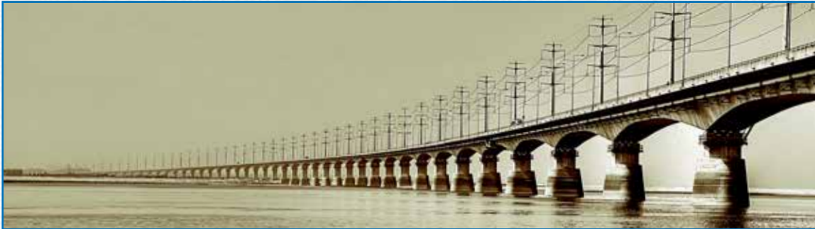
Bangabandhu Bridge on the Jamuna River
